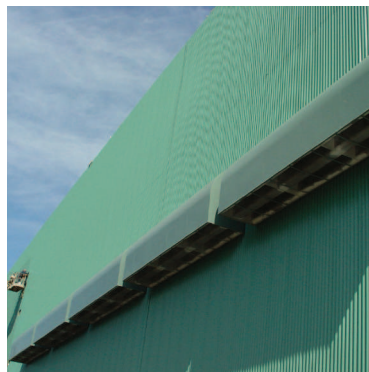
Intake Cowl Silencer for Gas Turbine Building Installation
